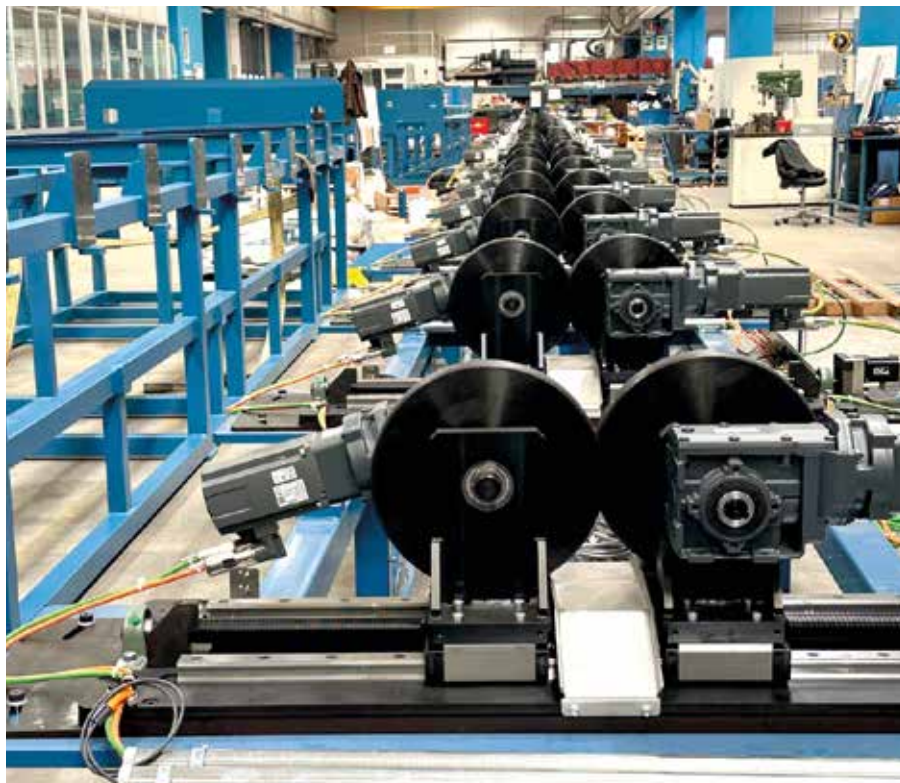
The new induction heat treatment line (under construction)
